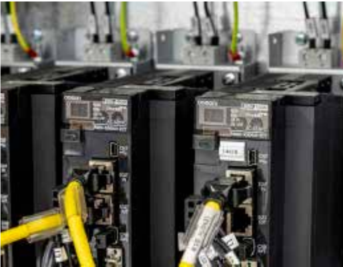
Omron servo drives and inverters ensure precise motion control and product positioning at exceptionally high operating speeds of up to 200 packages per minute.
